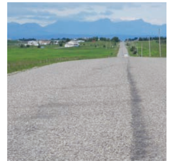
Road after TerraCem application
