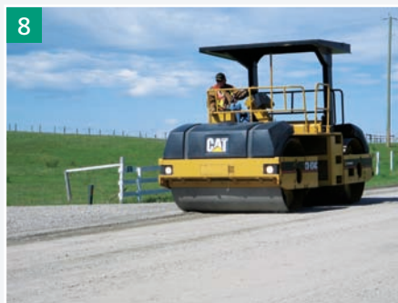
8 Smooth drum compactor for the final finish of the subgrade
