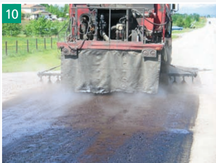
10 Oiling down a prime coat to keep the fines
