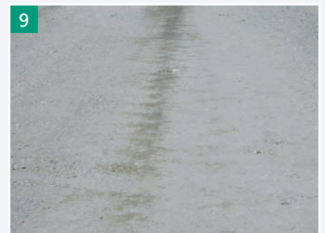
9 Finished subgrade now ready for surfacing
