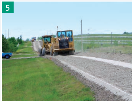
5 A grader follows the pulverizer to achieve homogenous mixing
