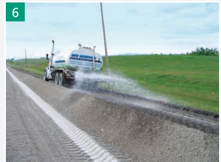
6 Addition of moisture to start the hydration process
