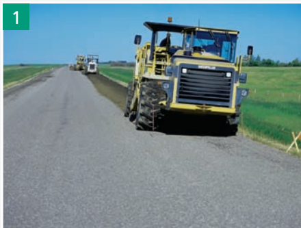
1 Pre-milling / pulverizing the existing road
