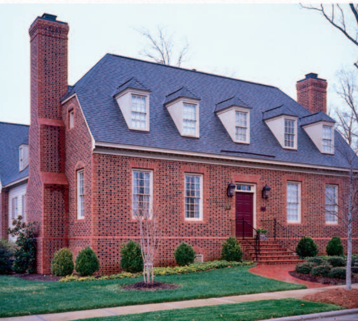
TOP Classic Williamsburg-style Colonial features slate roof, molded bricks and traditional mortar detailing.
