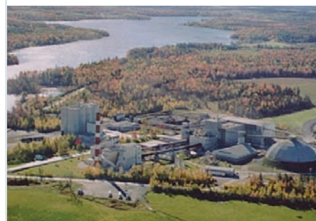
The Brookfield Plant is located north of Halifax, Nova Scotia and supplies well cements for the Hibernia Basin and Sable Island oil fields.
