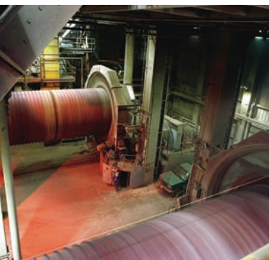
Large ball mills are used to grind the oil well clinker.
