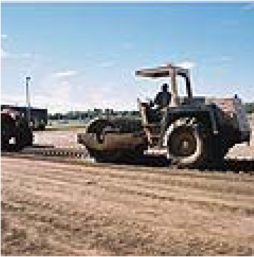
Compacting treated materials at Merrill Airport.
