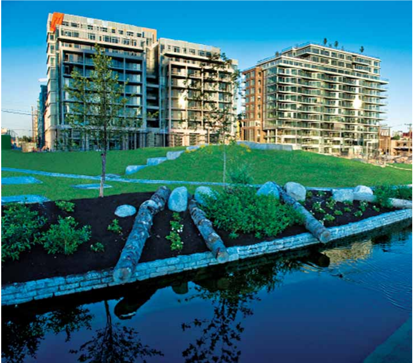
THE LEED GOLD VANCOUVER OLYMPIC VILLAGE USED LAFARGE'S FLY ASH IN THE CONCRETE TO HELP IT ACHIEVE HIGH STANDARDS OF ENVIRONMENTAL DESIGN.
