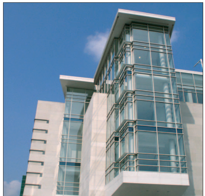
Also pictured on the cover, the Washington, D.C. Convention Center exemplifies the importance of properly produced, placed, finished, and cured concrete. Supplementary cementitious materials can avoid concrete failures, providing long-term performance with minimal maintenance.
