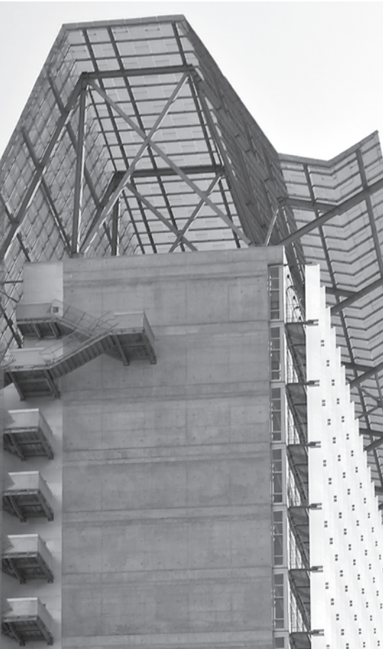
U.S. Federal Building San Francisco, CA
