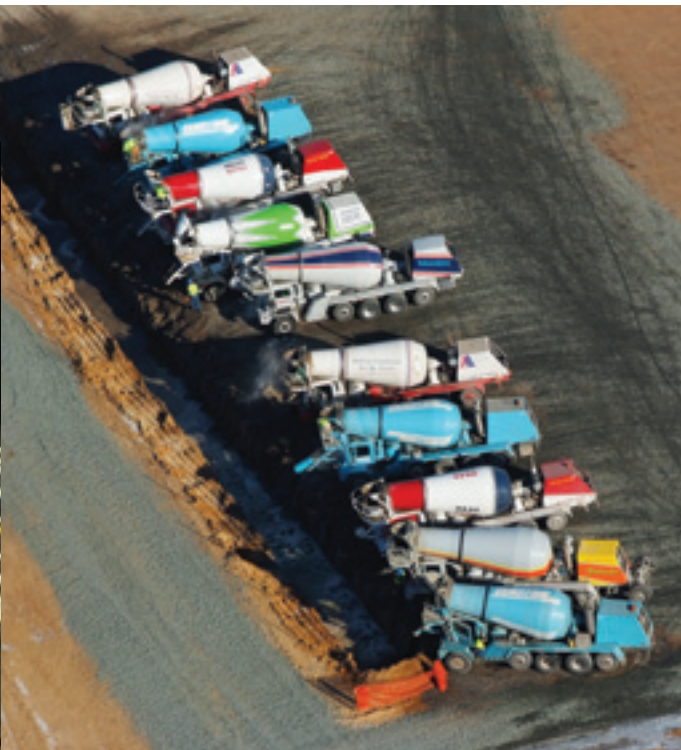
Measuring 168,939 cubic feet and holding more than 800 tons of steel reinforcement, the concrete slab at the Chippewa Falls, Wis., sand plant will support 12 silos, each 70 feet high and 48 feet in diameter.
